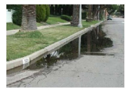
**DESCRIPTION:** This project provides for drainage improvements on streets with flat grades throughout the City. The work involves the reconstruction of curb, gutter, and pavement as necessary to correct drainage problems.
