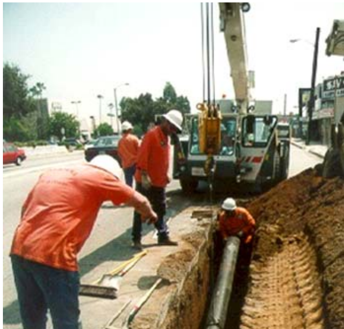
Fire Protection System Improvements
