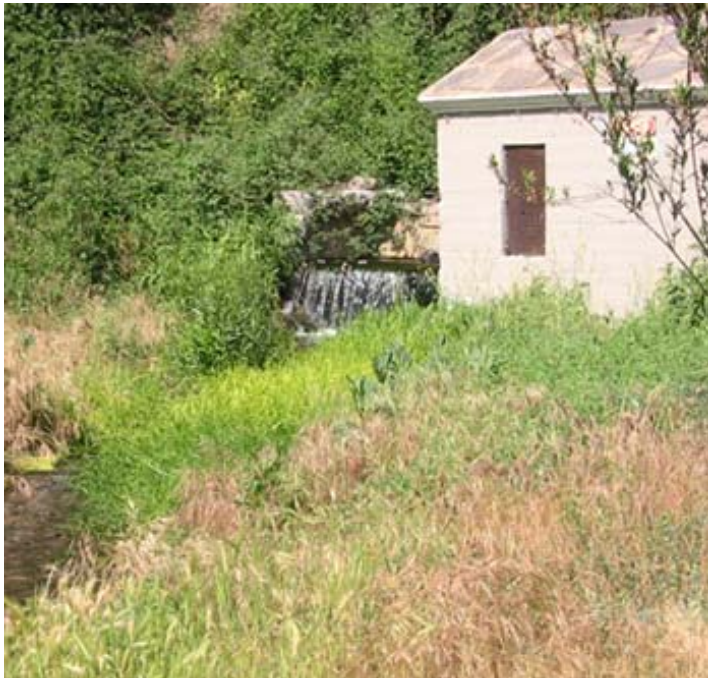
Water flow from Devil's Gate Tunnel
